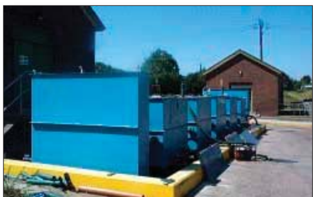
ABR installation. Photo courtesy of Atkins Water, 2006.
